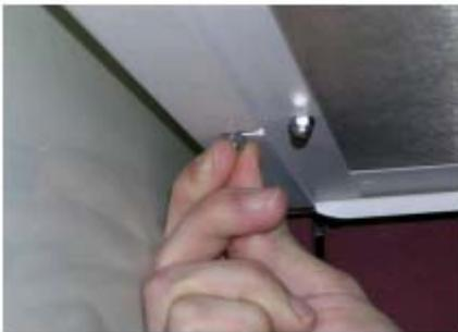
8. Remove the two acorn nuts that are located on the bottom of the drawer and set these aside to be used in step 12.
